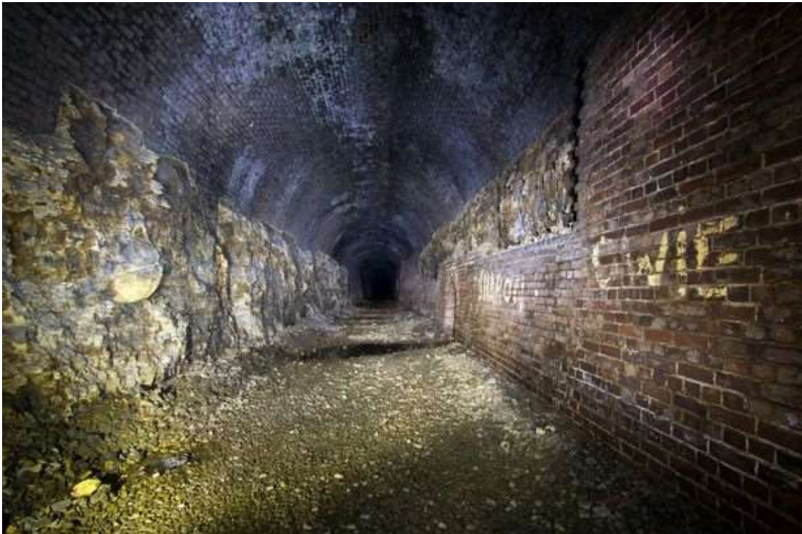
Inside the Abernant Tunnel (Image: Scott Lewis)
