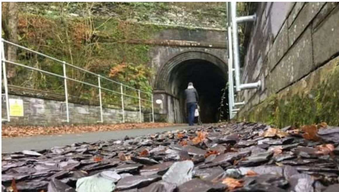
Tregarth Tunnel (Image: Gwynedd Council)
