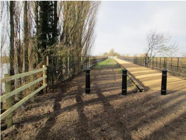
This photo shows the view west from the Torksey end and shows the new bollards installed to prevent vehicles access and the mesh panels fixed to the trestle viaduct parapets
