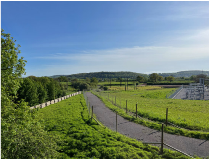
The soon-to-be-opened National Grid path at the new Hinkley Point Sandford substation, broadly following the railway alignment. This will replace the permissive path through Thatcher's orchards and the on-road section at Nye Road.
