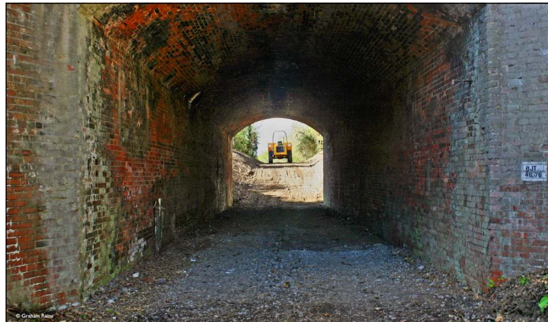
Clearance of Stourpaine tunnel.
