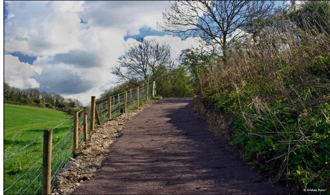
New access ramp from Mill Lane, Stourpaine.
