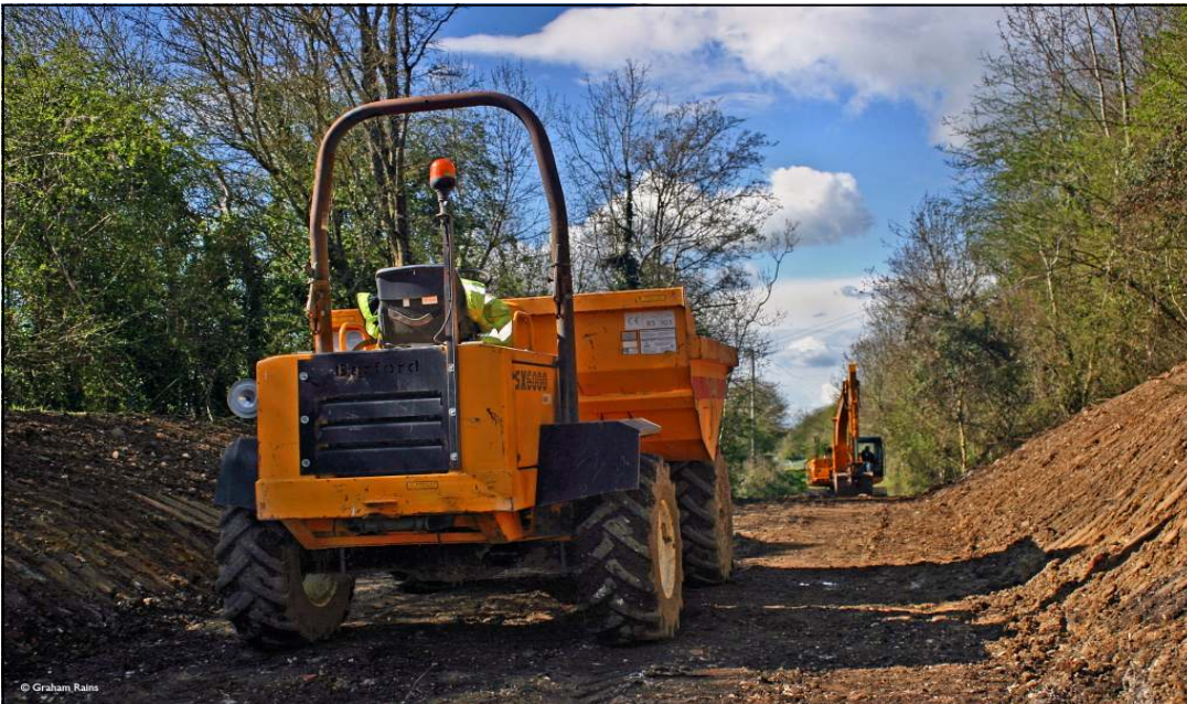
Construction of gradient to the north entrance of Stourpaine tunnel.
