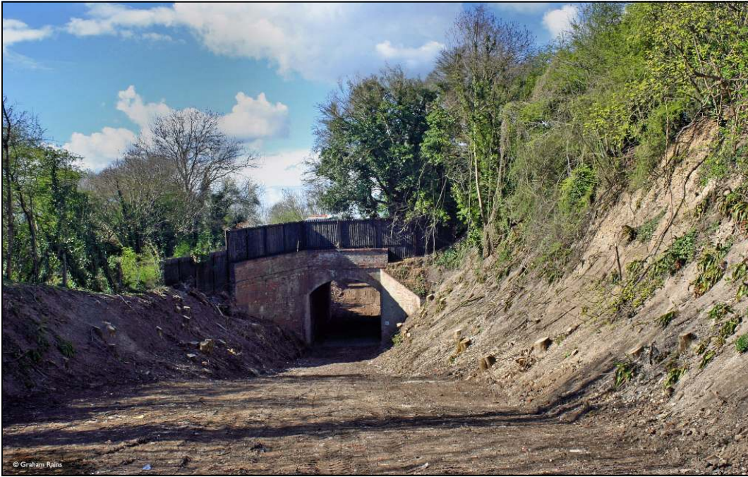
Gradient to south entrance of Stourpaine tunnel.
