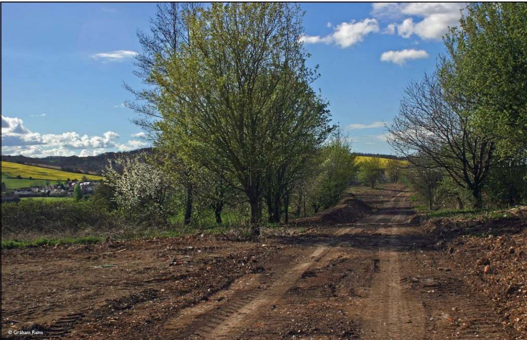
Section from Stourpaine tunnel, south to Manor France Farm crossing.
