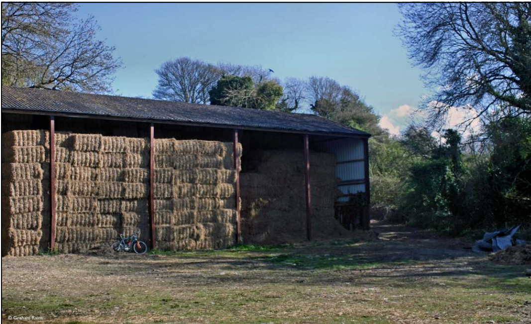
Barn situated on south side of bypass, to be re-sited.
