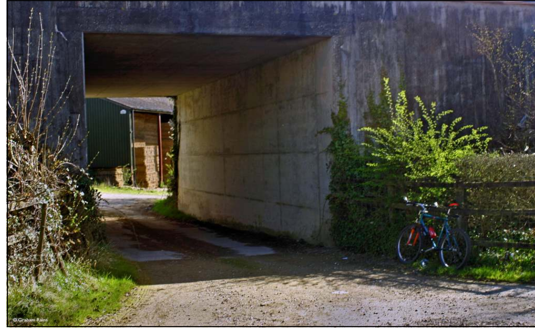
Underpass Blandford bypass.
