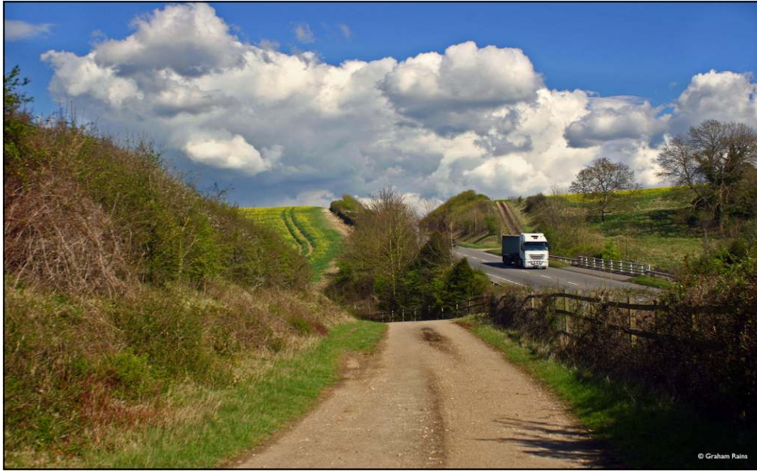
Underpass approach, north side of Blandford bypass.
