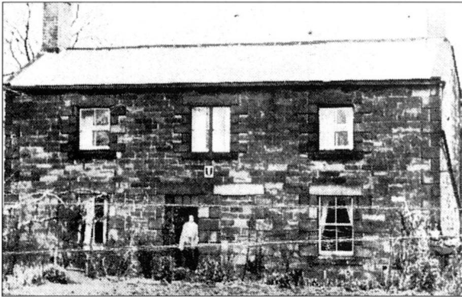
Etherley Engine-man's Cottage
